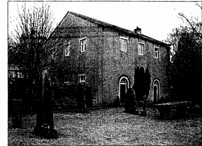
Chapel elevation (west) indicating wall bowing following outward roof thrust
